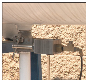
Internal excess flow valve
