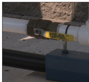
Ball valve in the open position
