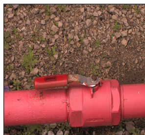
Ball valve in the open position
