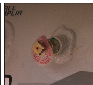
Fixed maximum liquid level gauge
