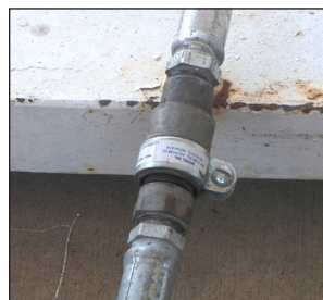
Emergency break-away device
