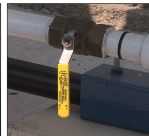
Ball valve in the closed position
