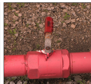
Ball valve in the closed position
