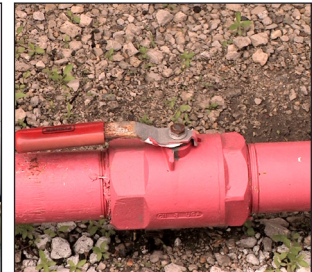
Valves controlling flow of propane
